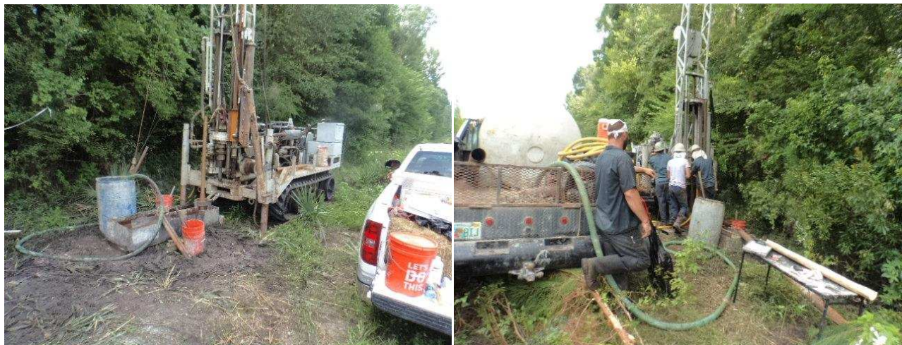
(Left) Track-mounted drill rig performing geotechnical drilling north of the Withlacoochee River. (Right) A second exploratory drill hole being performed along the HDD alignment, north of the Withlacoochee River.
