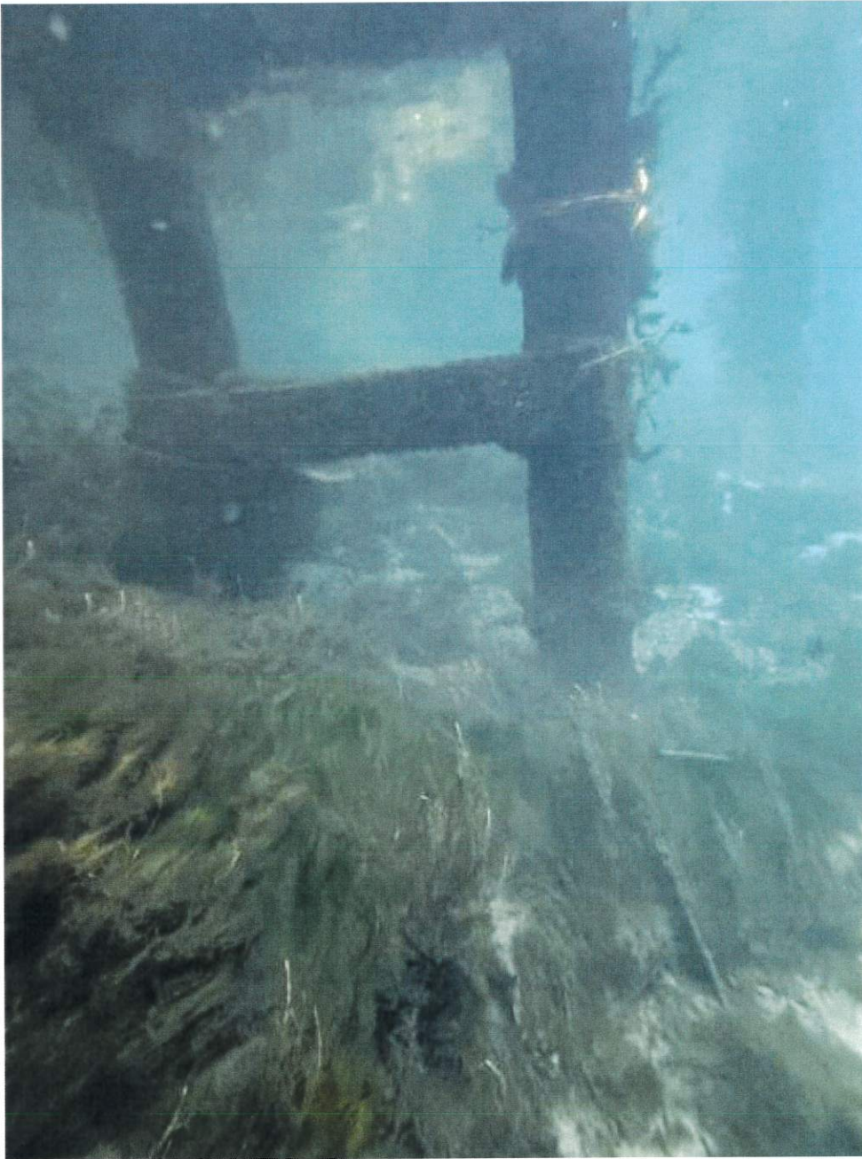
Figure 2: 09/06/2025. Submerged aquatic vegetation primarily consists of filamentous algae. Loss of soil around pilings beneath private dock at 218 SW Riverside Ave, Fort White, FL.
