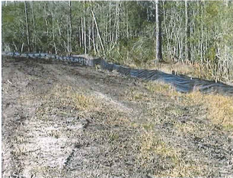
Silt Fence Repaired (January 31, 2024)
