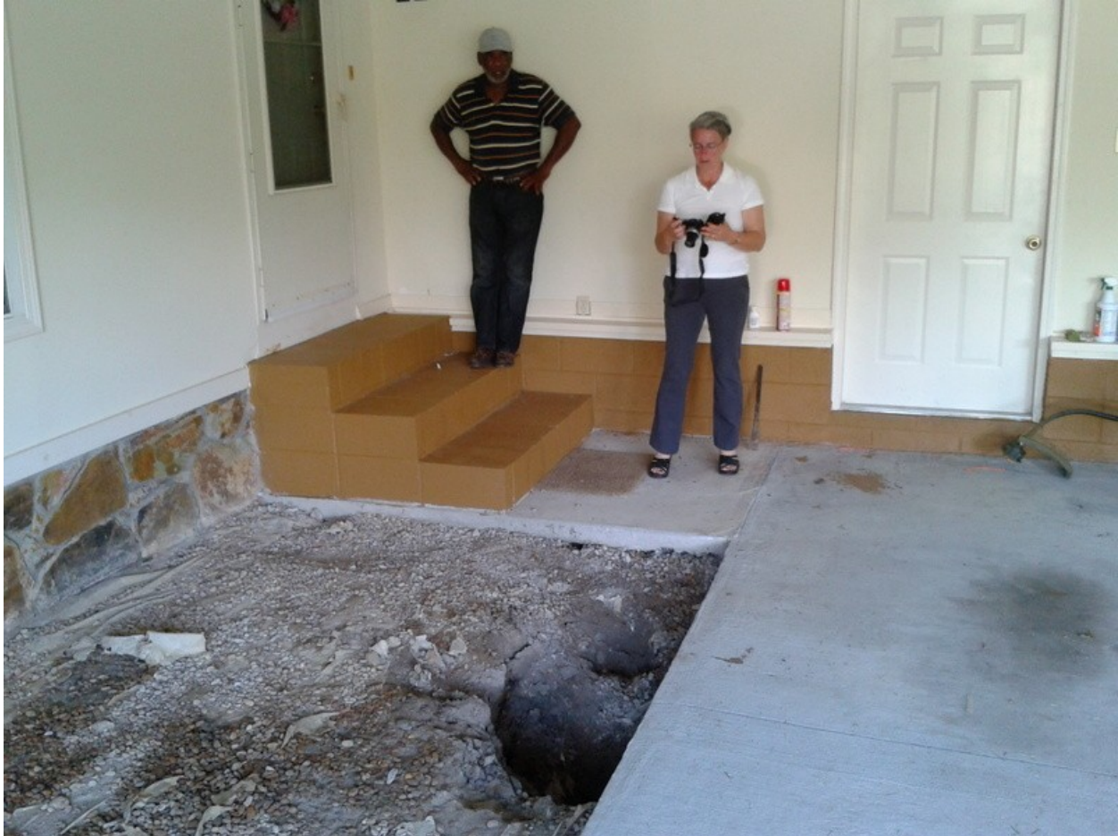
Illustration 5: Exhibit D-- Sinkhole under a garage in Lowndes County, Georgia.
